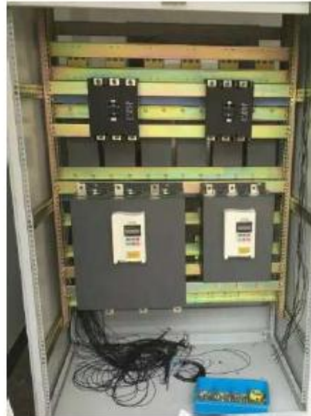
On line soft starter which working no need by pass contactor
