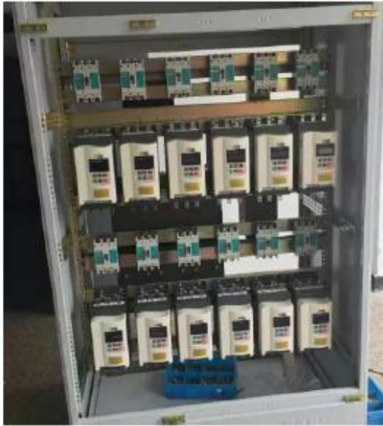
On line soft starter which working no need by pass contactor
